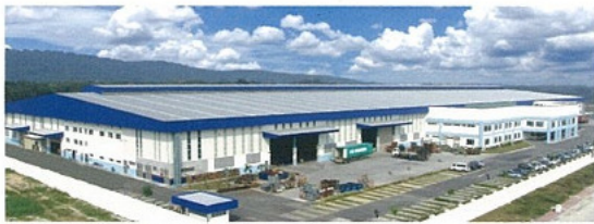
Plant at Kota Damansara, Selangor
